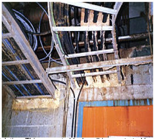
Code Violation: This concrete block wall is penetrated by cable trays and cables. The hole should be fire stopped to restore the fire-resistance rating of the wall. Instead, it is filled with flammable polyurethane foam
